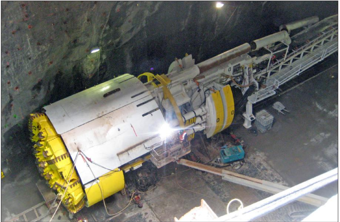
Hard Rock TBM 1
