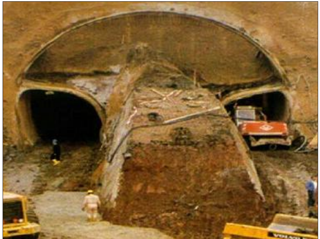
SEM Operation at a Tunnel Portal 2
